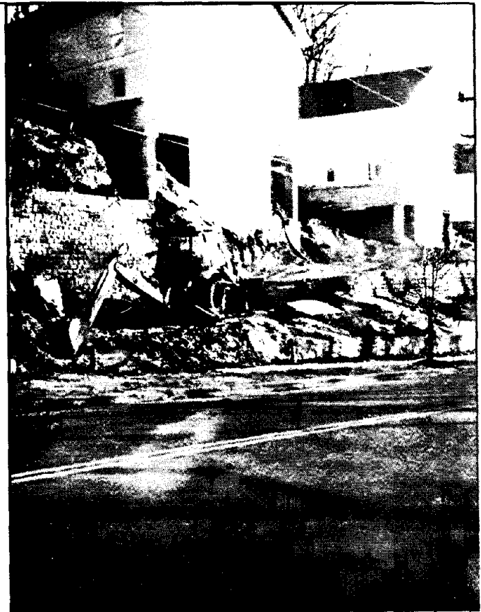
Rain washes loose dirt from this construction site down a steep city hill into a stream at the bottom.
