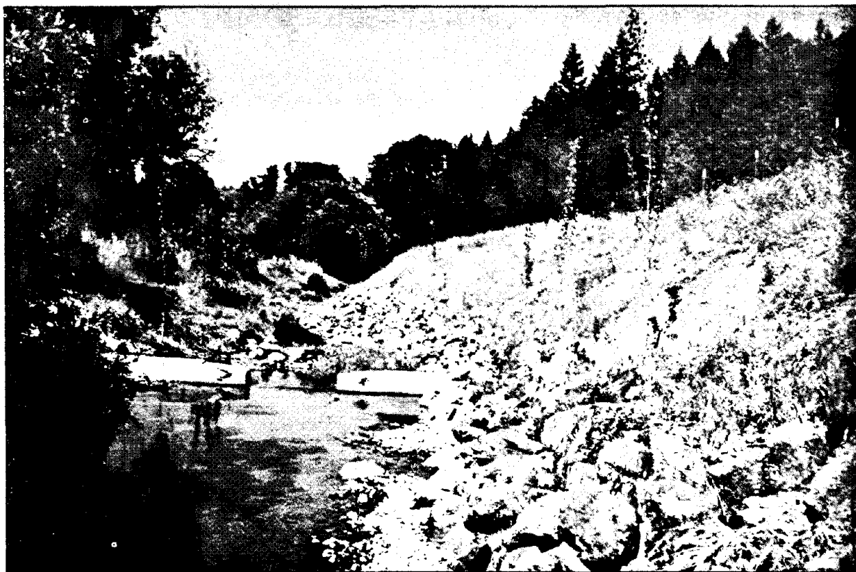
Rock riprap retains the soil on this slope above a creek.
