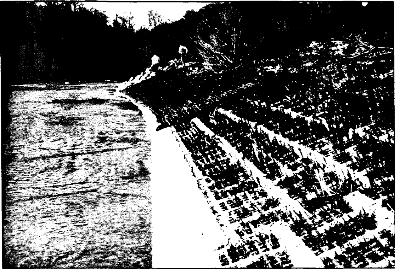
Vegetation has been plugged into this slope to prevent erosion.
