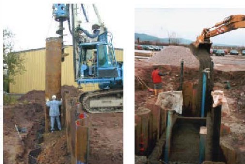
Figure 3 – Right photo: set-up of the vertical drainages using a large diameter borehole construction method; left photo: filling the gate with \text{Fe}^0
