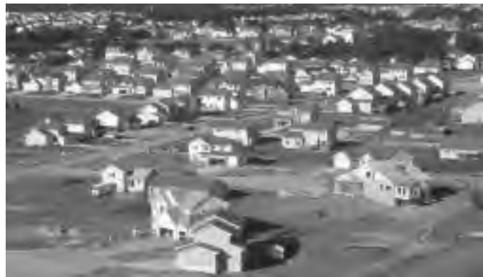
This building site in Dallas County, Iowa, represents many low-density development practices.
