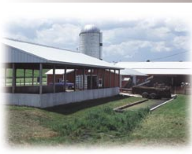
Roofed and concrete wall solid manure stacking facility with a settling basin and filter strip.
