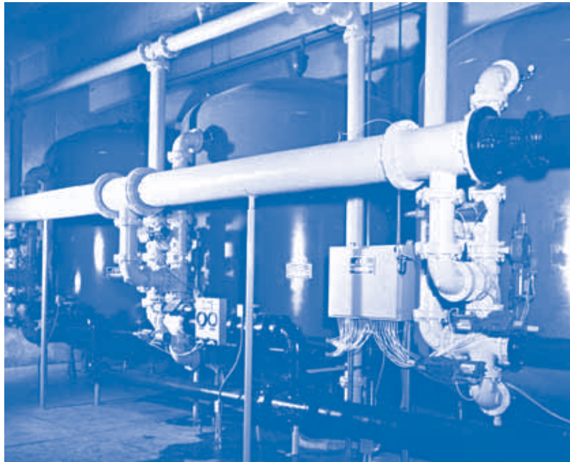
Figure 6-6. Ion Exchange System (Tonka Equipment Company).
