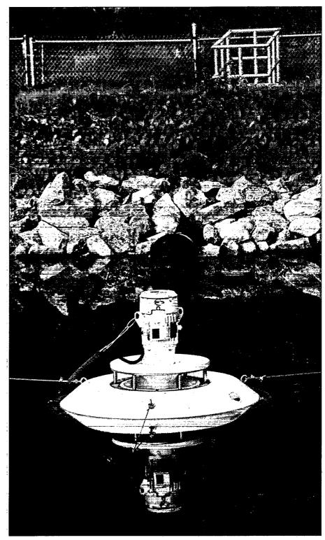
reduced the financial impact of the upgrade on the community and provided it with a system that would require only slightly more maintenance than the existing stabilization pond. Post-aeration is essential for compliance with the effluent standard for dissolved oxygen.
