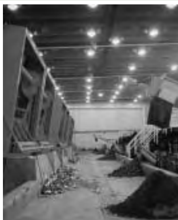
Photo: Trash screens at Atlanta's Intramural Creek CSO Center. Courtesy of Atlanta Department of Public Works
