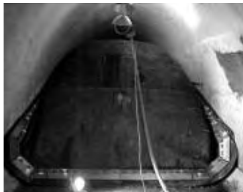
Photo: Inflatable dam at the Sneads Branch CSO. Courtesy of LJCMSD
