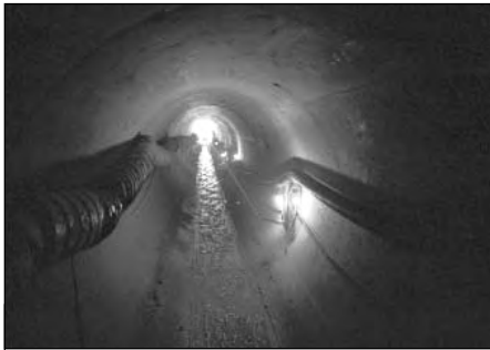
Sewer separation tunnel installed by New Brunswick, NJ. Sewer separation is the most common long-term control used by CSO permittees.
