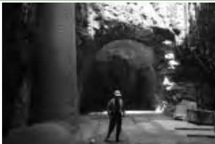
Photo: Construction of a 6.7 million gallon storage tunnel along the Falls of the James. Courtesy of Richmond DPU
