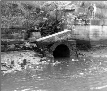
Addressing deteriorating infrastructure, such as this crumbling CSO outfall, is one aspect of most CSO control programs.
