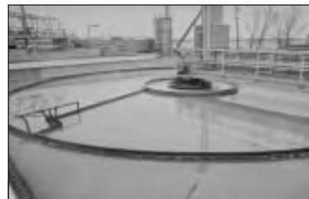
Like most cities, Chicago maintains excess primary treatment capacity to accommodate wet weather flows. Shown is a primary clarifier at a Chicago-area POTW.
