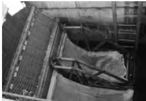
Photo: Solids and floatables controls, such as the nets pictured here, are installed at all North Bergen CSOs. Courtesy of NJDEP
