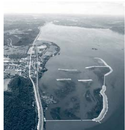
Pool 8 Island Complex 99 Aerial
