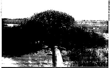
The discharge from the hydraulic dredge pumps a slurry of bottom sediments onto the face of the marsh.
