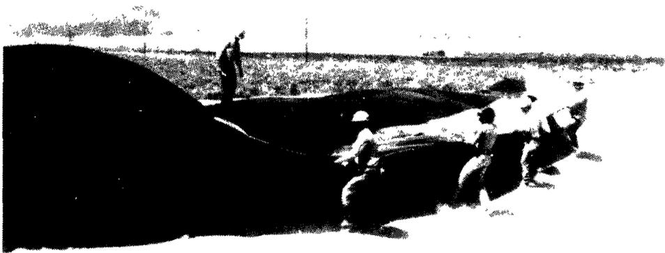
Figure 9-23. Workmen "pulling" a panel fabricated from a fabric-reinforced FML across the subgrade. This step can be difficult to accomplish during windy conditions.
