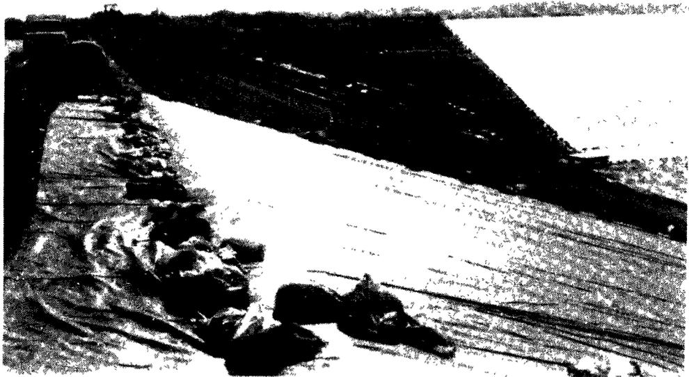
Figure 9-15. Use of sandbags to anchor unseamed sheets and unseamed edges of FMLs to prevent wind damage.
