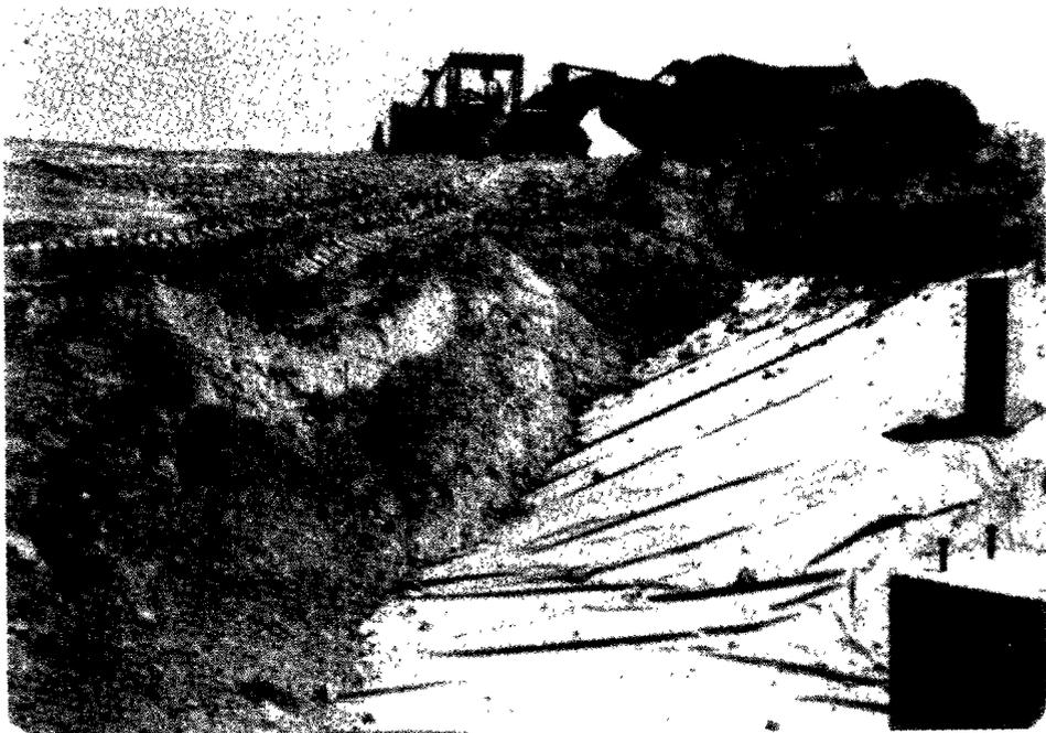
Figure 9-2. Trenching machine for anchor trenches (top). Dozer and earth mover for berm construction (bottom).
