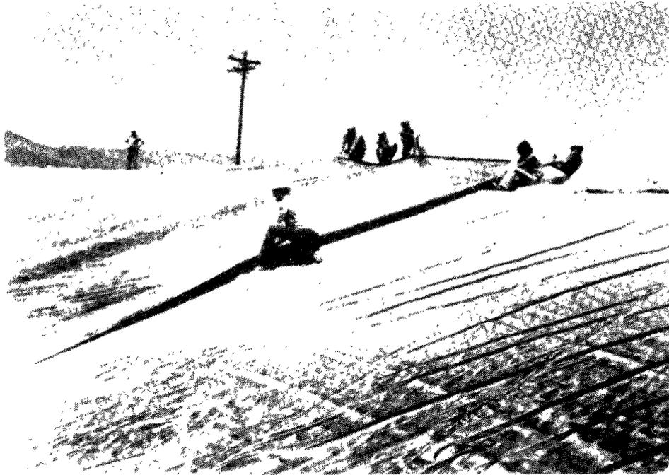
Figure 9-25. Pulling an FML panel smooth. Each FML panel must be pulled smooth, leaving enough slack to accommodate anticipated changes in dimensions due to temperature changes.
