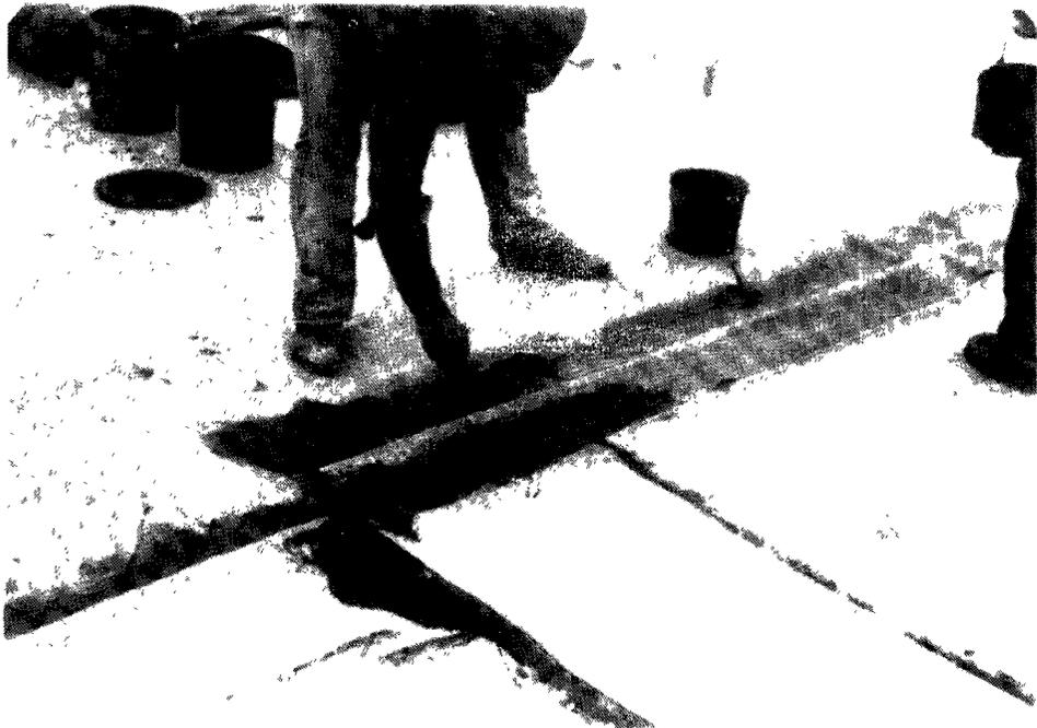
Figure 9-30. Field seaming of a fabric-reinforced thermoplastic FML using a solvent-based technique. The bodied-solvent adhesive is applied using either a squeeze bottle or a paint brush.
