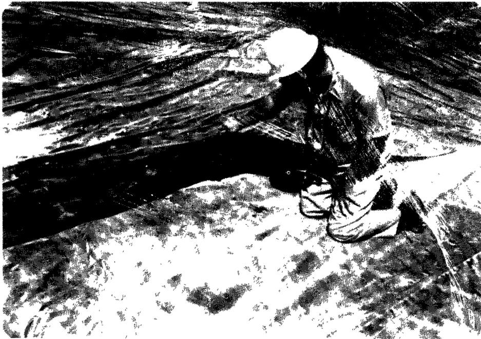
Figure 9-27. Inspecting overlap between panels of a fabric-reinforced FML. Sufficient seam overlap must be maintained. Manufacturers usually specify minimum overlap for field seams.
