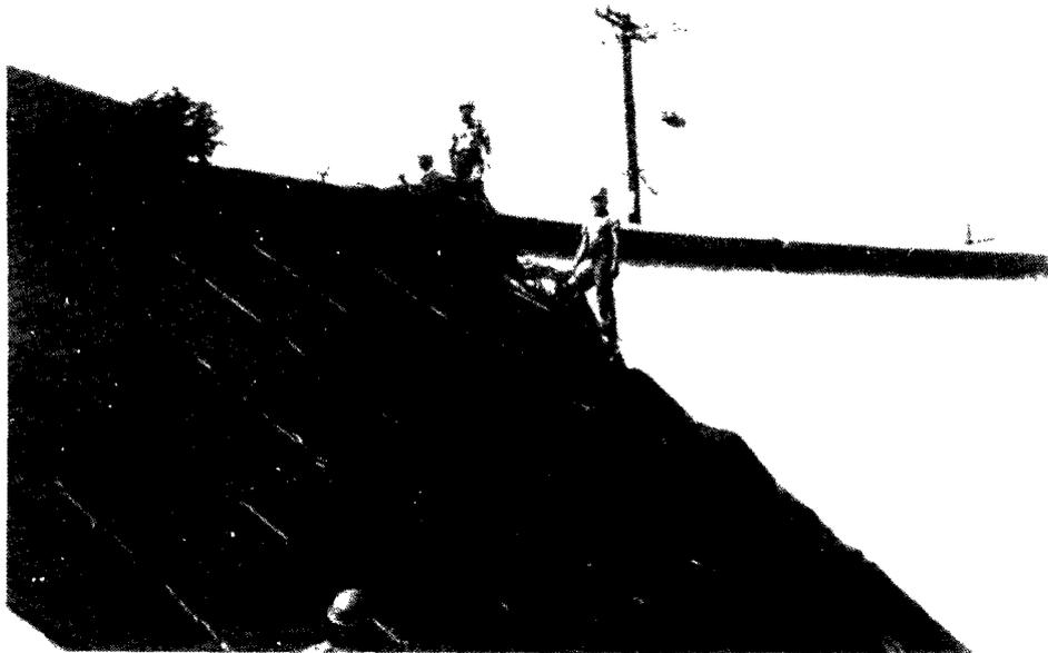
Figure 9-24. Spotting a panel fabricated from a fabric-reinforced FML. Once an FML panel has been unfolded, the crew "spots" or positions it in the proper location.
