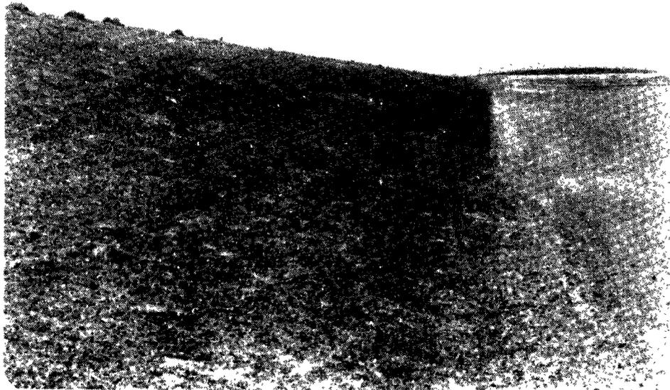
Figure 9-10. Representative subgrade surface texture prior to placement of an FML.
