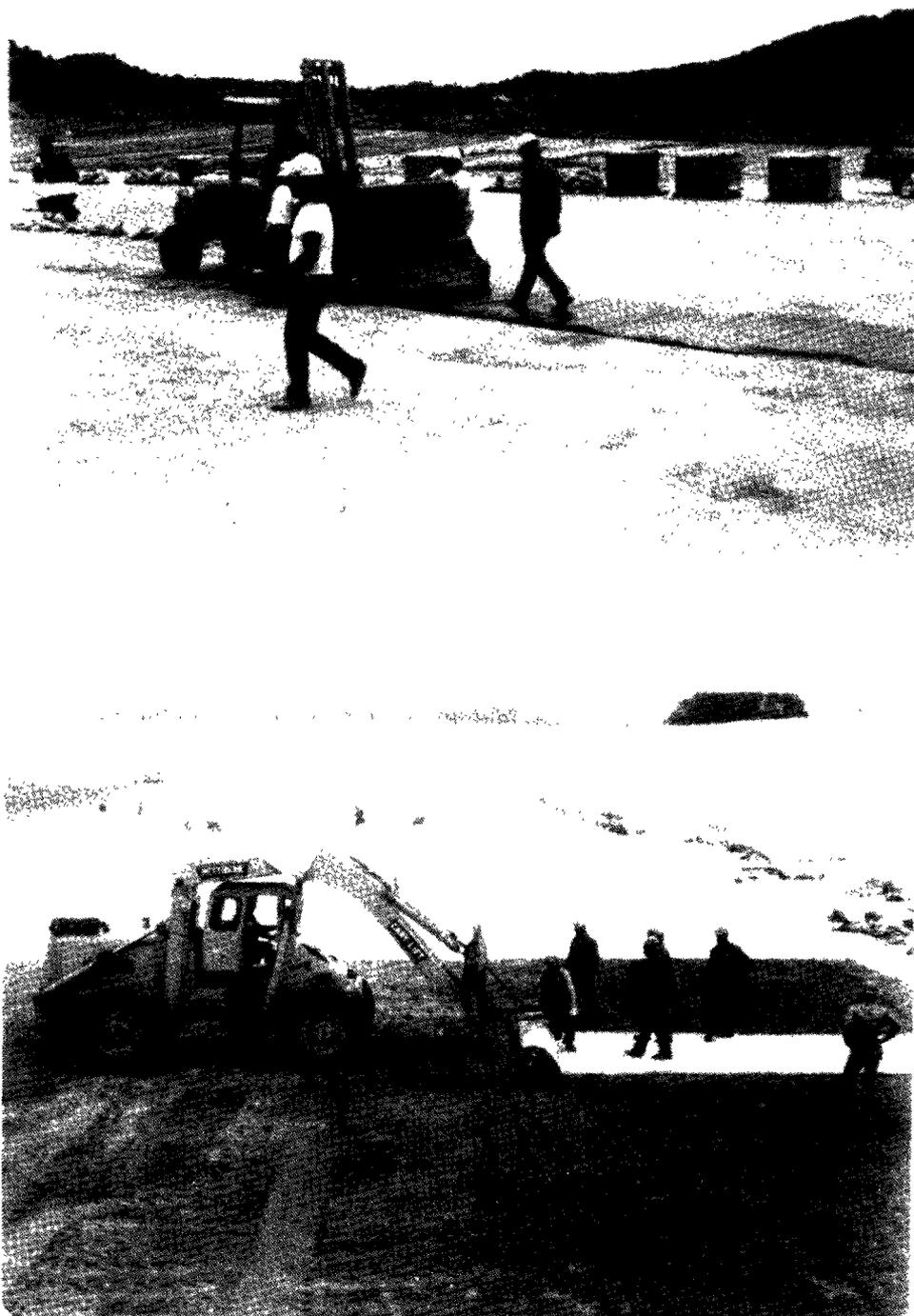
Figure 9-22. Panels of a fabric-reinforced FML being unfolded or unrolled.
