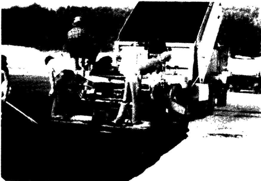
Figure 9-38. A 2-in. thick asphalt concrete liner being applied using road paving equipment and methods. After the surface cools, a seal coat is applied (Source: Shultz, 1982).
