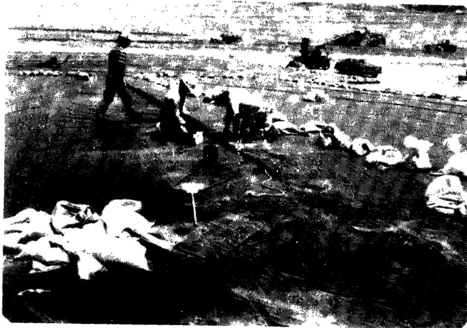
Figure 9-19. Field seaming operation using bodied-solvent adhesive. A board is being used for support under the area being seamed; the board is pulled along under the seam with the rope shown in the picture.
