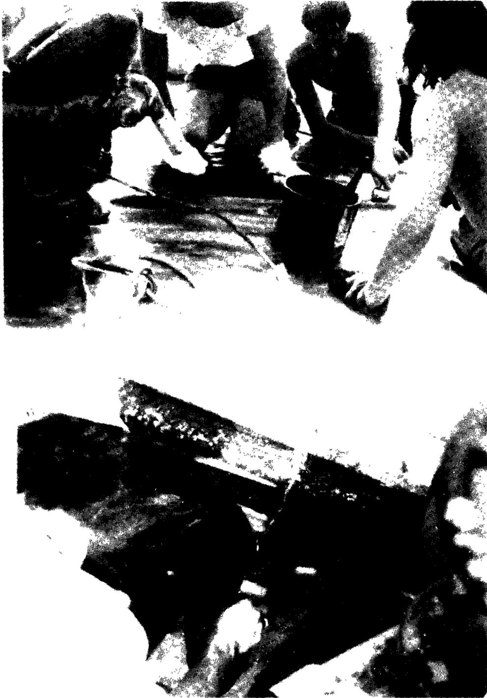
Figure 9-20. Heat guns being used to facilitate field seaming of FMLs.
