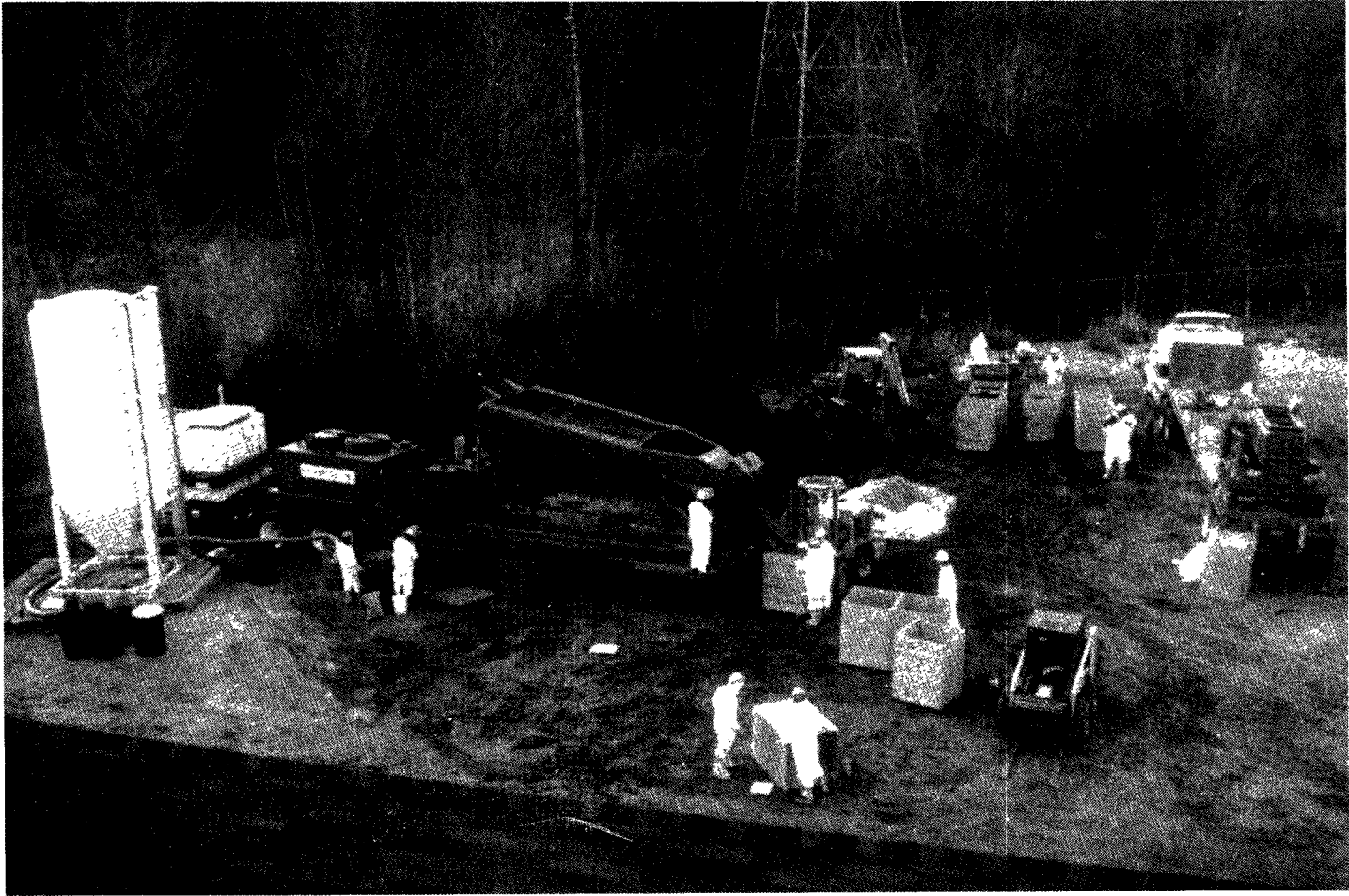
Figure 2. Overview of the Soliditech demonstration in progress
