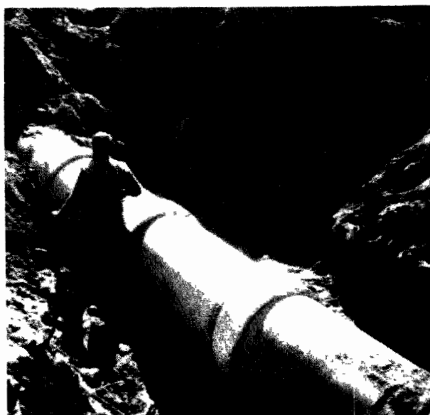
Figure 38. Repair in break of mainline pipe, 1 meter diameter
