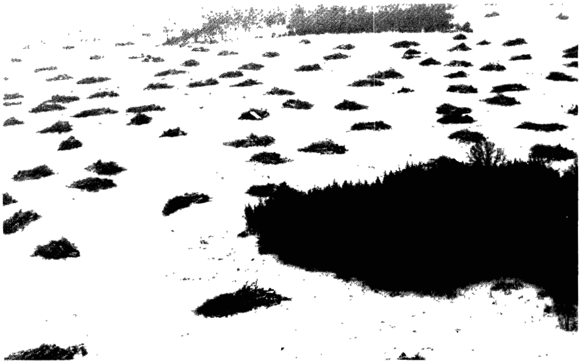
Figure 7. Stacks of bulldozed trees in early clearing operation
