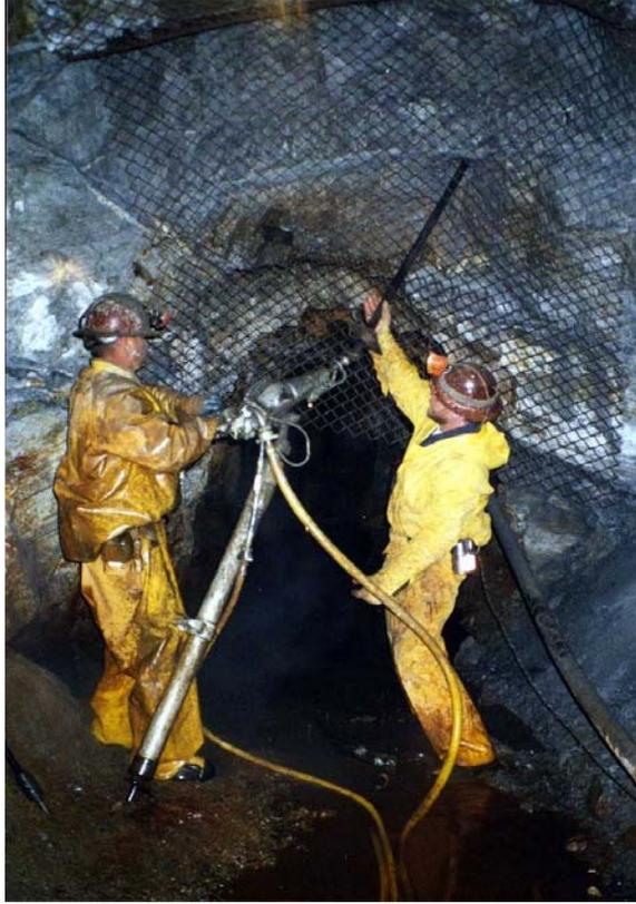
**Figure 5-1. Stabilizing the underground mine working of the Miller Mine with roof bolts and screen using a Gardner-Denver Model 83 Jackleg drill.**
