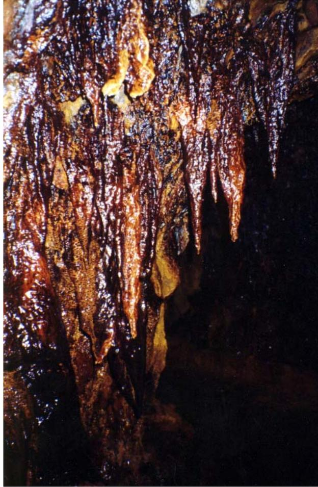
**Figure 5-3. Iron oxide stalactites in the W1 drift, which were areas where flow through the fractures required grouting.**
