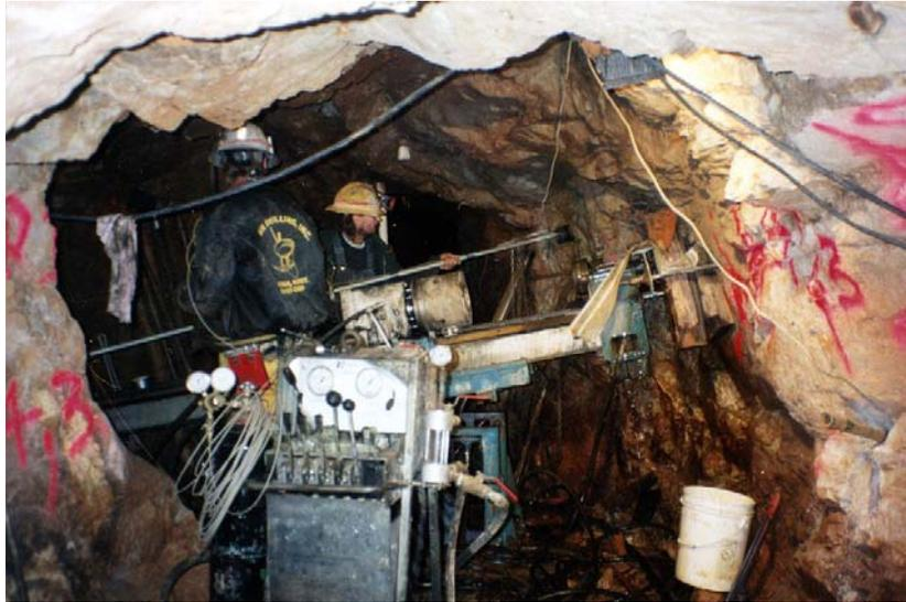
**Figure 3-1.** The drilling/gROUTING subcontractor placing an inflatable packer system into the grout hole for dye and water injection testing.
