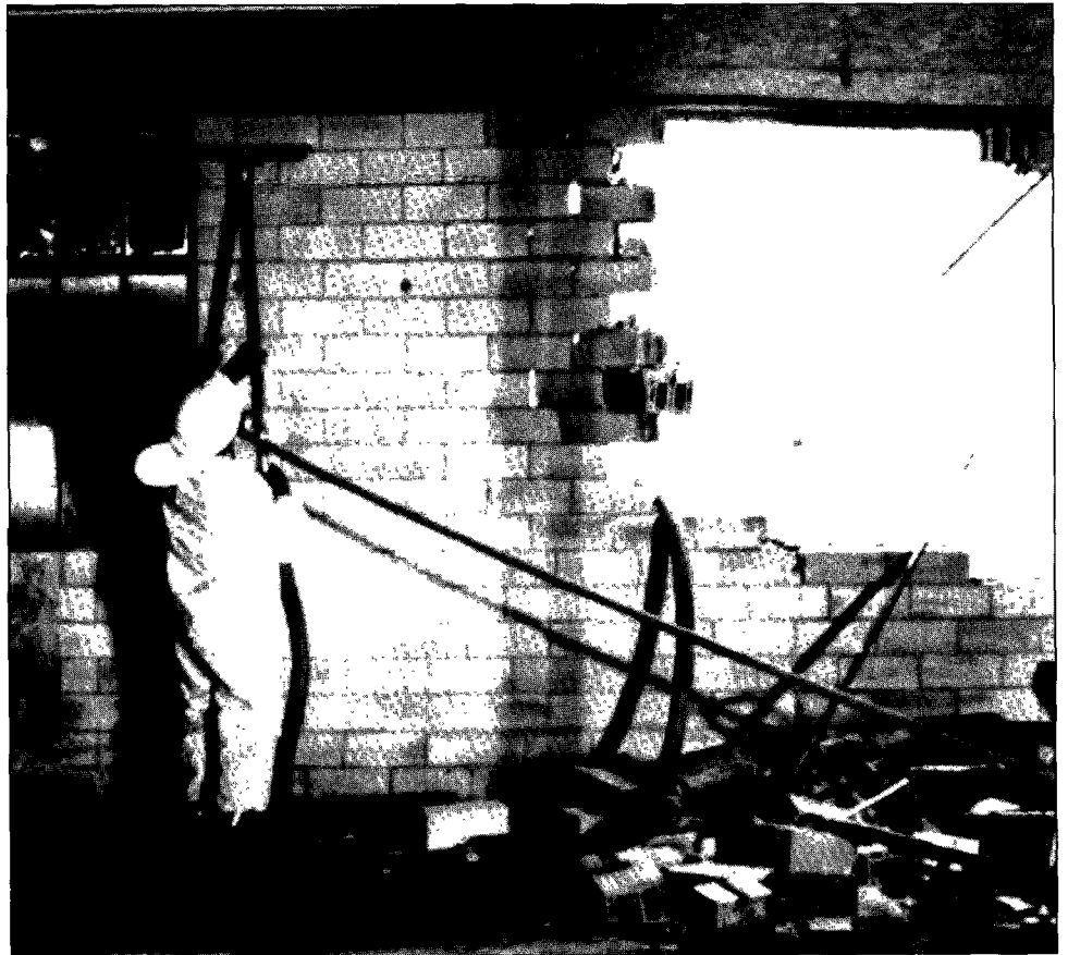
Decontamination at Tri-State Plating: the main processing building was decontaminated and its foundation excavated. Walls were blasted with abrasives, then residues removed by high-power vacuum.
