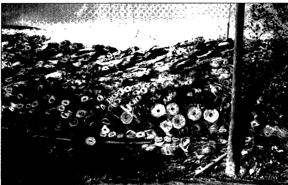
Pipes, shingle rolls, and manufacturing waste were used to build up the side walls of a 33-acre settling basin where asbestos fibers formed a sludge.
