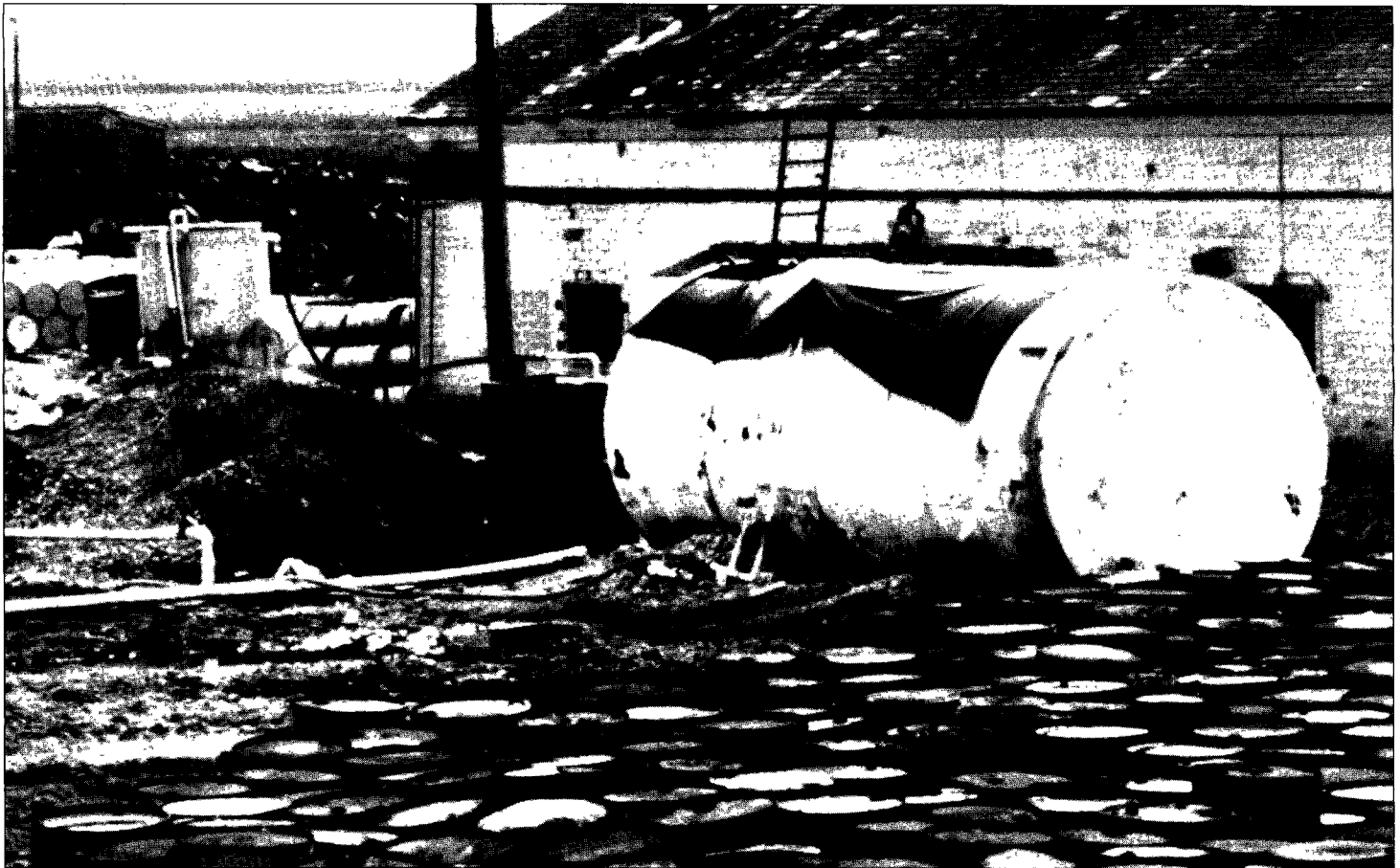
Solvents, acids, and heavy metals from leaking barrels polluted soil and ground water over a 12 - year period.
