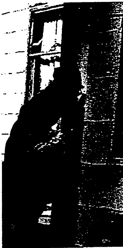
Volunteers for Christmas in April wear masks as they scrape peeling lead-based paint from their designated home.
