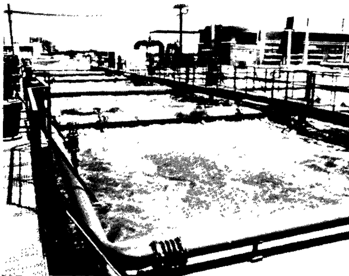
Activated Sludge Aeration Tank
