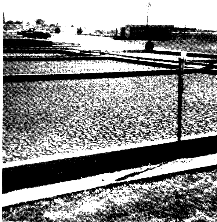
Sludge Drying Bed
