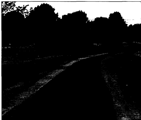
This walking path at the Earvin “Magic” Johnson Recreation Area in Los Angeles County is made from rubberized asphalt, which is more resilient than traditional asphalt.
