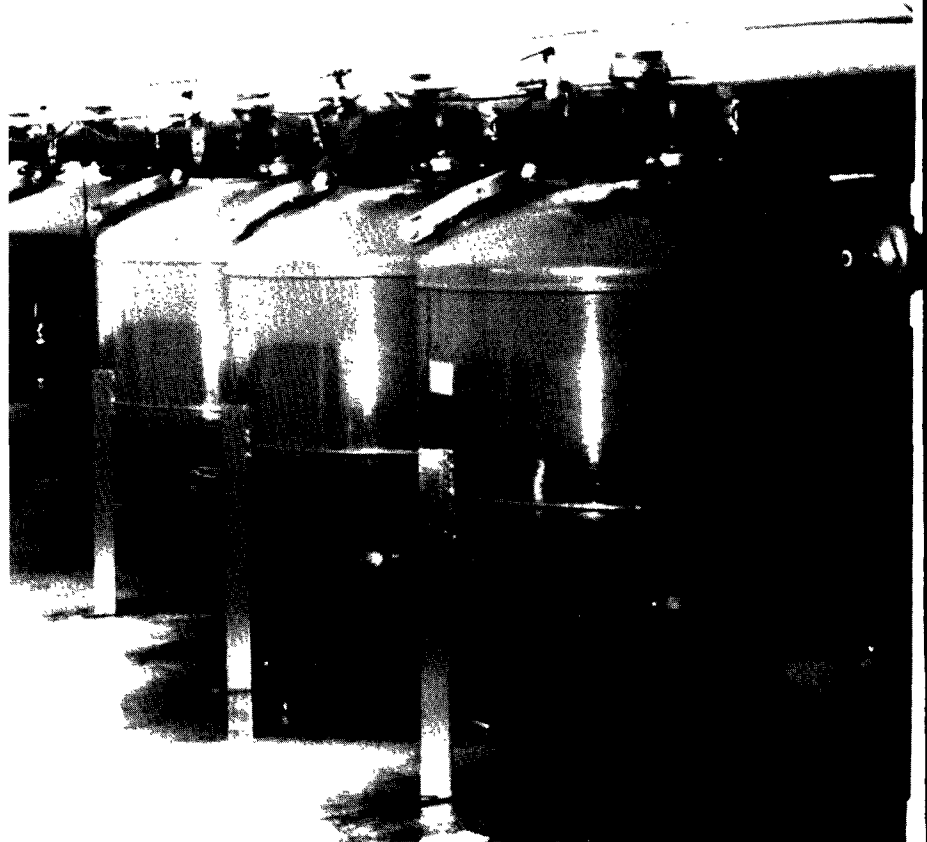
Sand filters for water treatment at Hines Nursery near Houston, Texas.
