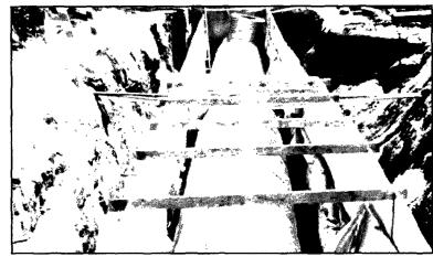
Exfiltration trenches with pipes, fabric wrap and rock are being used in central Florida. From these operating systems, it was concluded that the treatment volume should not be placed in the water table. In southern Florida, the pipe is frequently not used; however, the systems must be maintained to remove debris. Maintenance will vary directly with the amount of debris.
