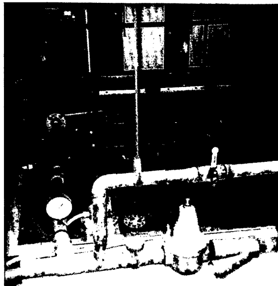
FIGURE 6. Crane Microstrainer
