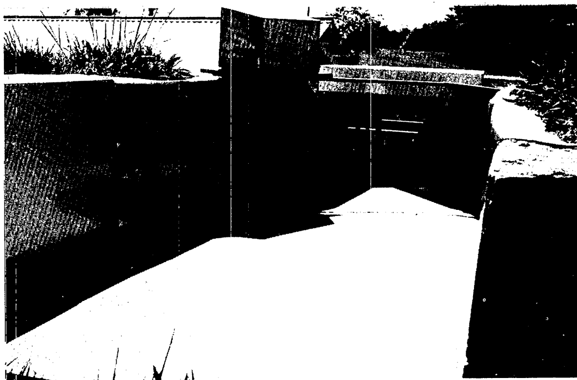
FIGURE 3.14. H-type flume with sloping floor approach.
