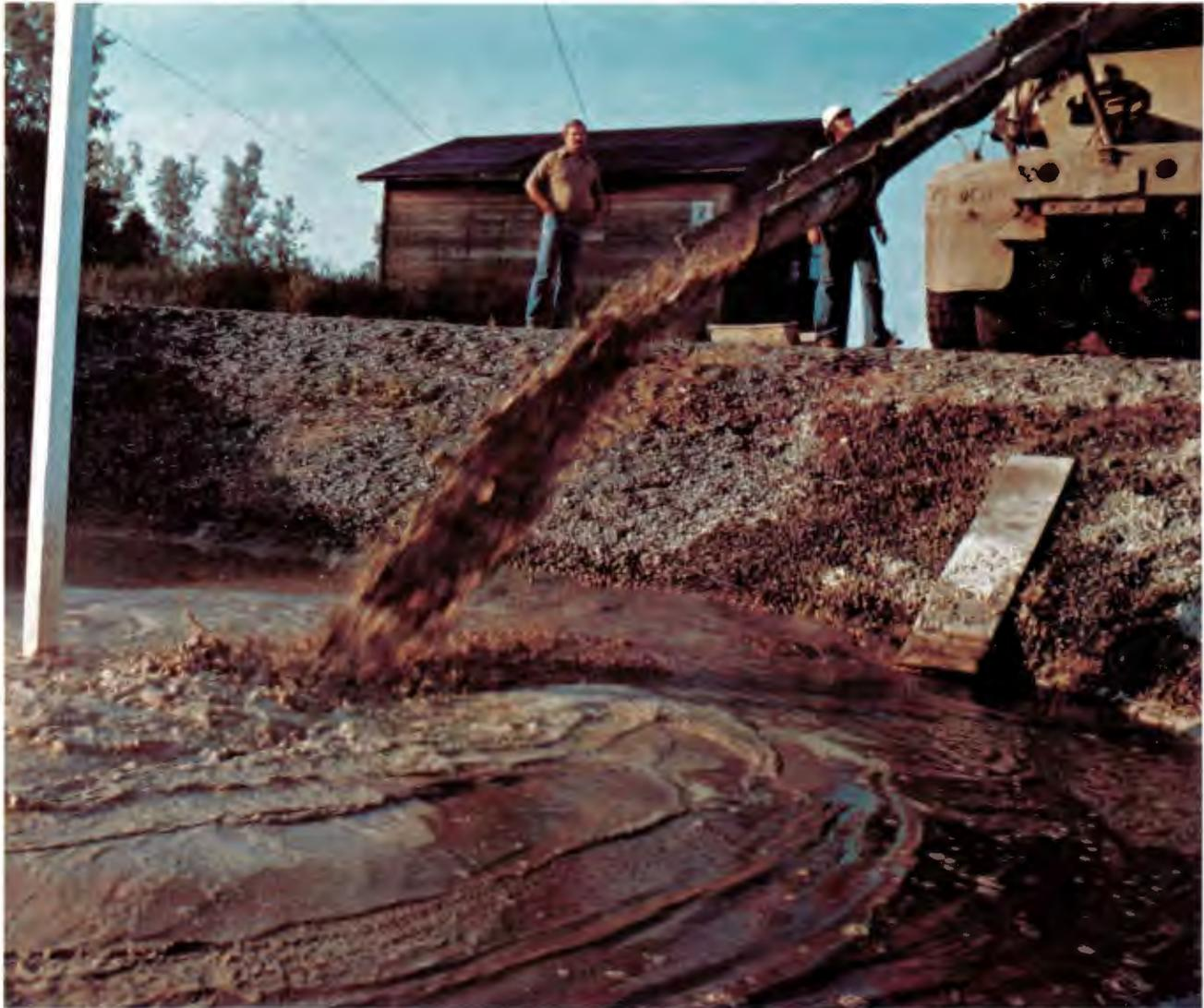
Filling lower portion of Site H with scrubber clarifier underflow slurry that has been force-oxidized to gypsum
