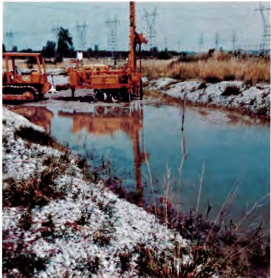
Chemically treated Site E, containing trapped water, supporting drilling rig during waste coring operation
