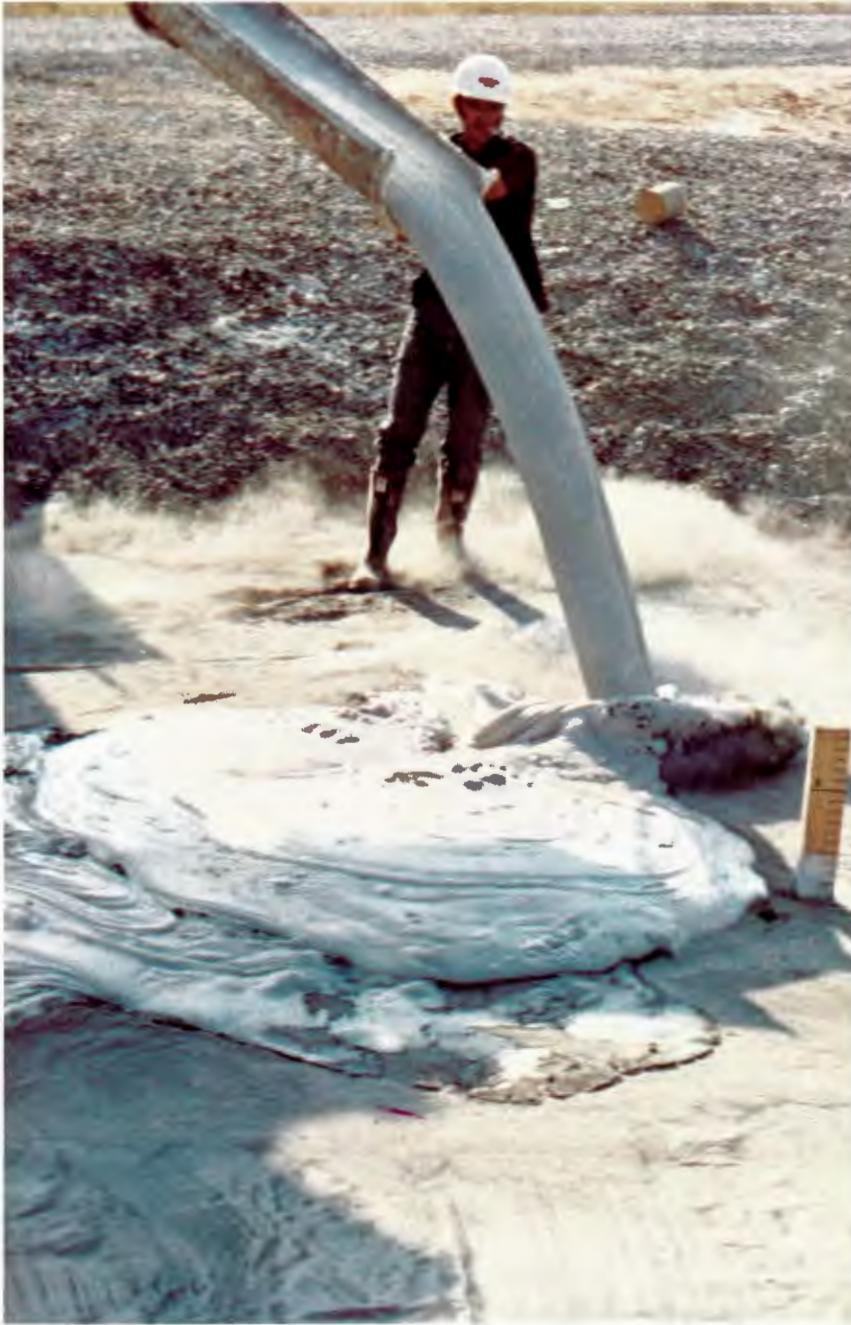
Untreated underdrained Site G supporting personnel during filling operation
