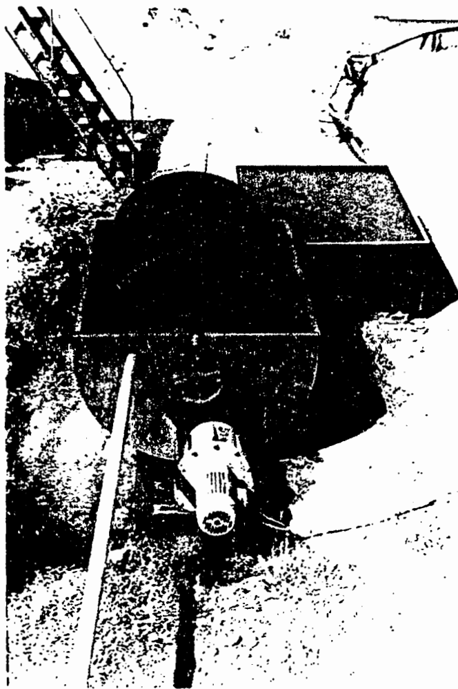
Photograph : 1 Rotating Biological Contactor showing Biological Slime on Discs.
