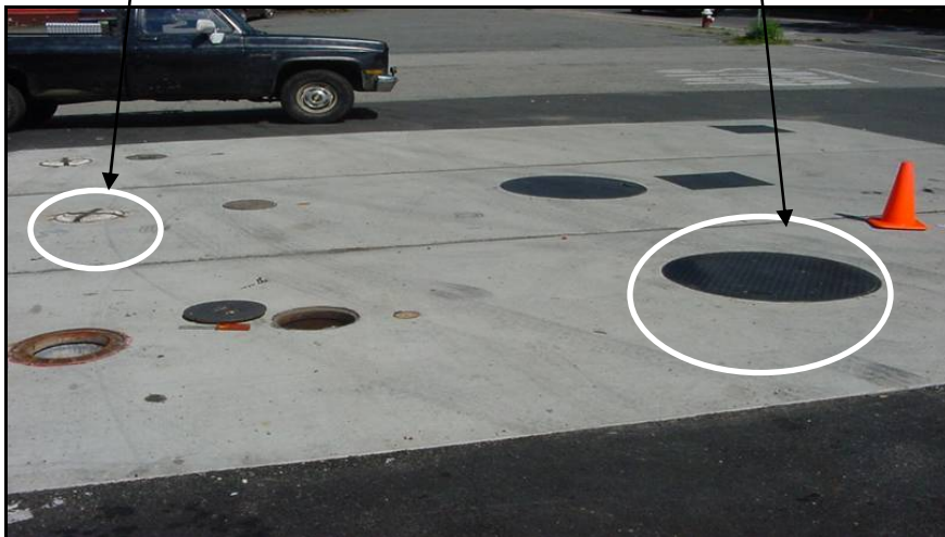
View of sump lids
