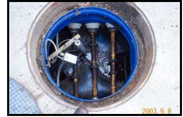
Transition/intermediate sump
