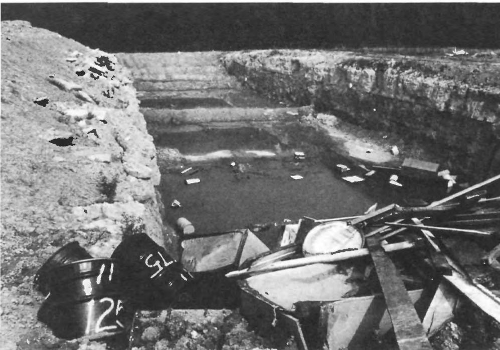
*Citizen concern led to the closure of and clean-up plans for the Maxey Flats low level radioactive waste site in Kentucky. Starting in 1963, nuclear waste had been buried in 51 trenches like this one.*
