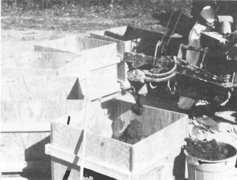
*HAZCON Solidification Process: Contaminated material is mixed with Portland cement, a patented additive, and water. Mixture hardens into a cohesive mass that immobilizes contaminants.*
