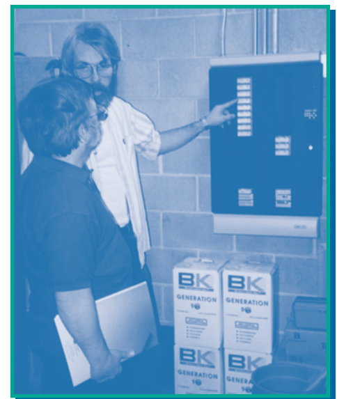
Rick Anderson, of Saint Paul's Environment and Energy Resource Center, looks on as John Benjamin, of the Public Works Department, describes an infrared heating system that saves money and reduces CO 2 emissions.
