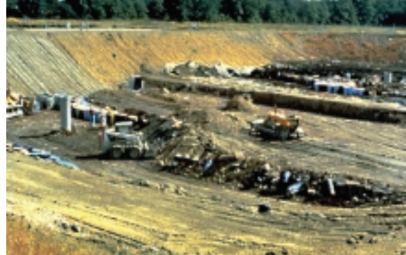
Here, personnel use heavy equipment to remove contaminated soils from a site.
