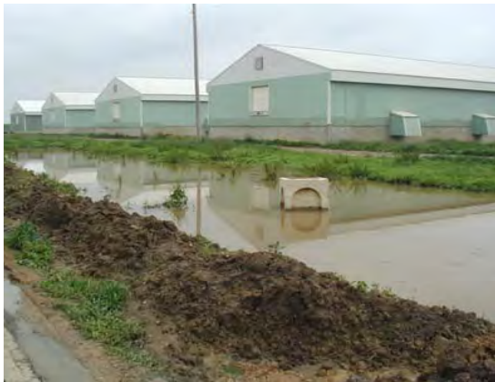
Poorly maintained facility affects storm water management.
