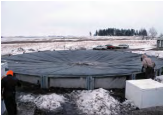
Dairies may use methane recovery systems to reduce air emissions and as an alternate energy source.
