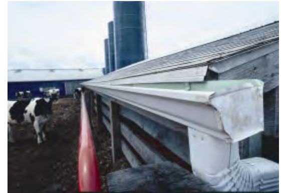
Gutters separate clean and dirty water and prevent water from accumulating in corrals.
