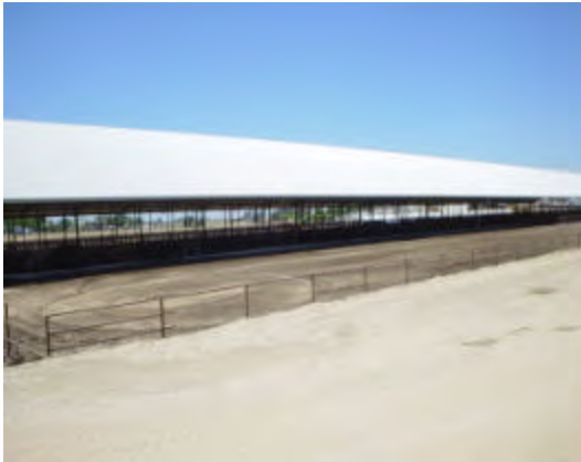
Covered livestock holding areas minimize the mixing of stormwater with manure and help keep the animals cool.
