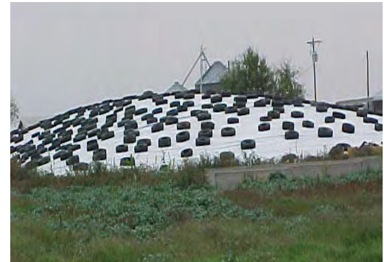
Bermed, secured, and covered silage prevents runoff.
