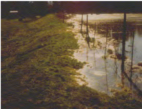
Overflowing manure storage pond has exceeded capacity.
