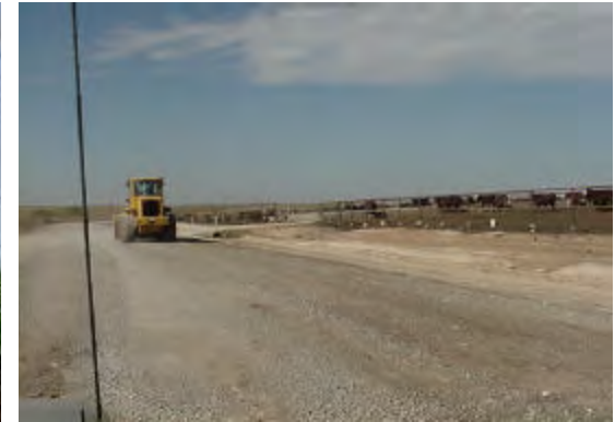
Cleaning solids from ditches allows effluent to flow freely to retention ponds.
