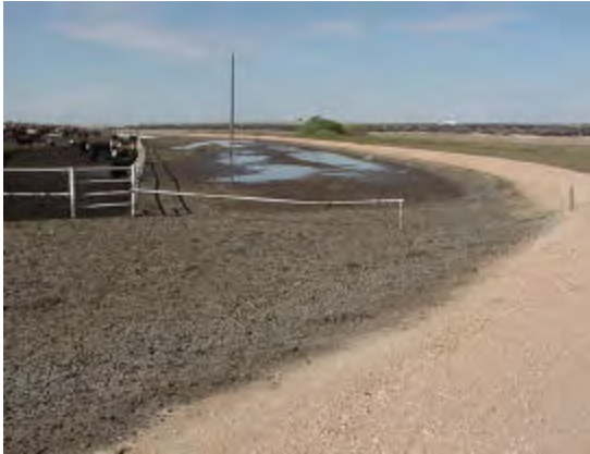
A bermed feedlot contains polluted runoff.
