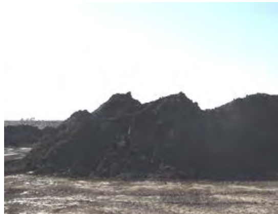
Runoff from unprotected stockpiles could pollute surface water.
