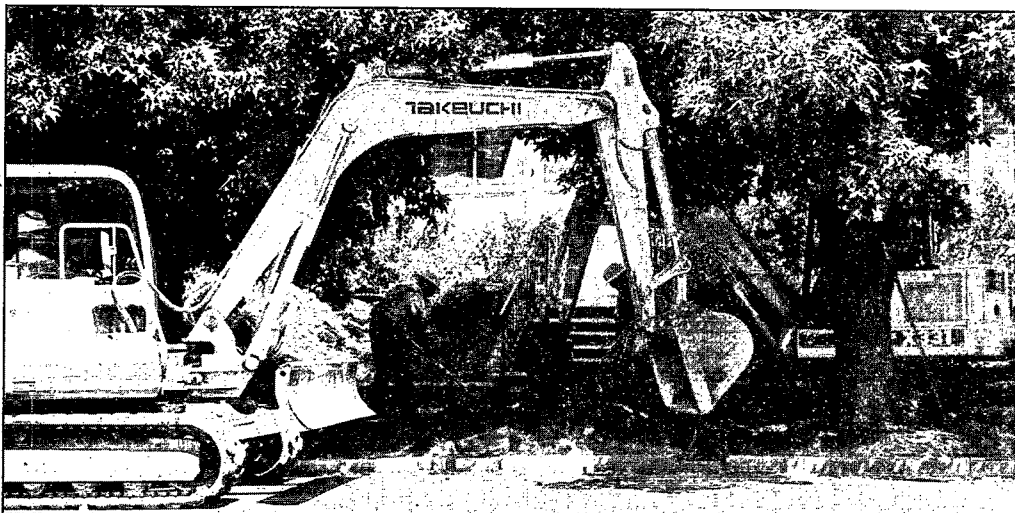
EPA will excavate and replace lead-contaminated yard soil at over 2,500 residences over the next five years.
