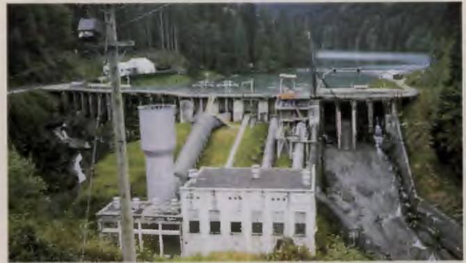
Figure 5.8: Elwha Dam. Fish passages were not constructed when the dam was built in 1910–1913.
