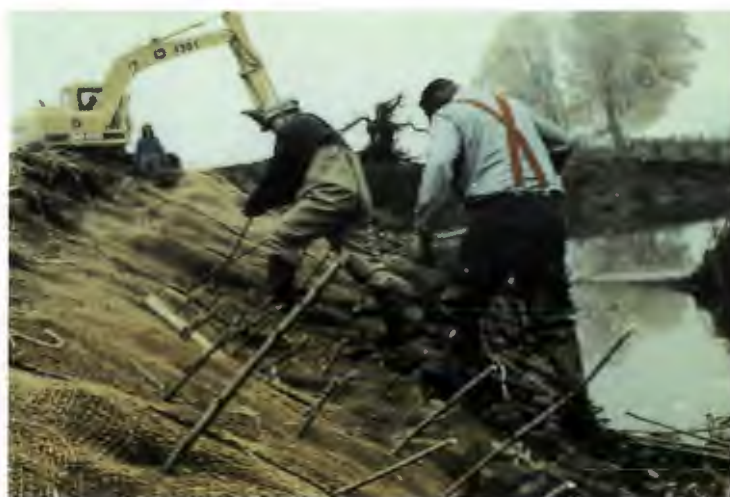
Figure 6.7: Installation of erosion control fabric. Installing measures can be considered a "mid-point" in restoration and not the completion. Preceding installation is the necessary planning, with monitoring and adaptive management subsequent to the installation.
