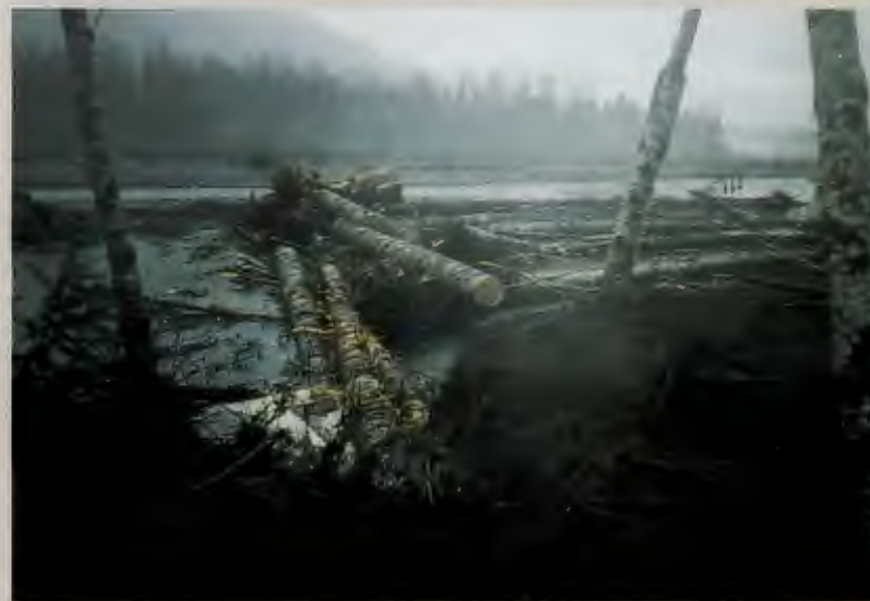
Figure 9.23: Engineered log jams. Engineered log jams (ELJs) can restore riverine habitat and in some situations provide effective bank protection.
