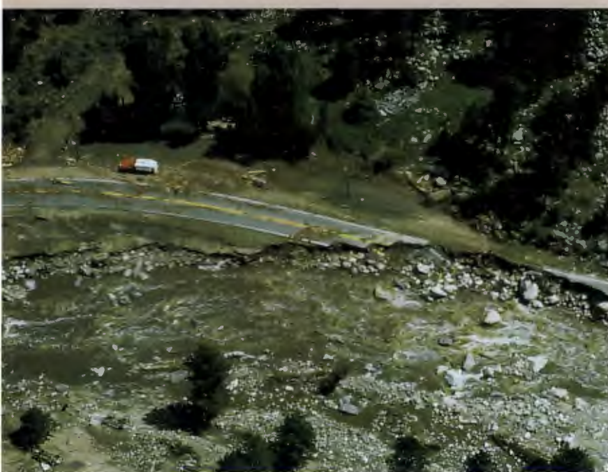
Figure 4.12: Bank erosion. The cause(s) of bank erosion should be identified.
