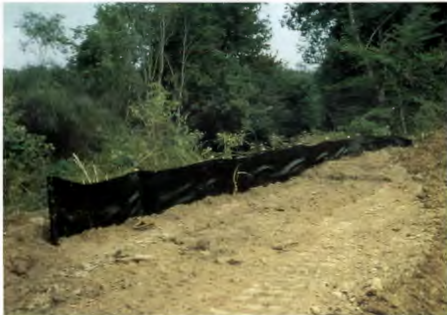
Figure 9.2: Silt fence at a construction site. Properly chosen and installed silt fences can provide a significant degree of off-site sediment control.
