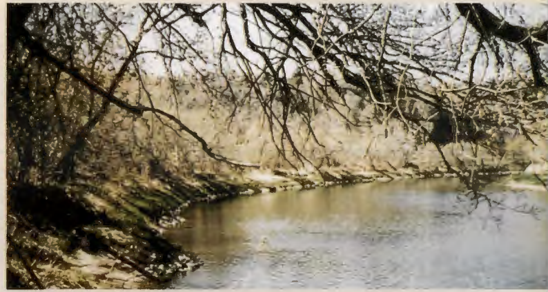
Figure 6.13: Same site (Figure 6.12) in April 1995. Note remnants of old jetties and heavy bank cover. Restoration measures are continuing to function well, more than 55 years after installation.
