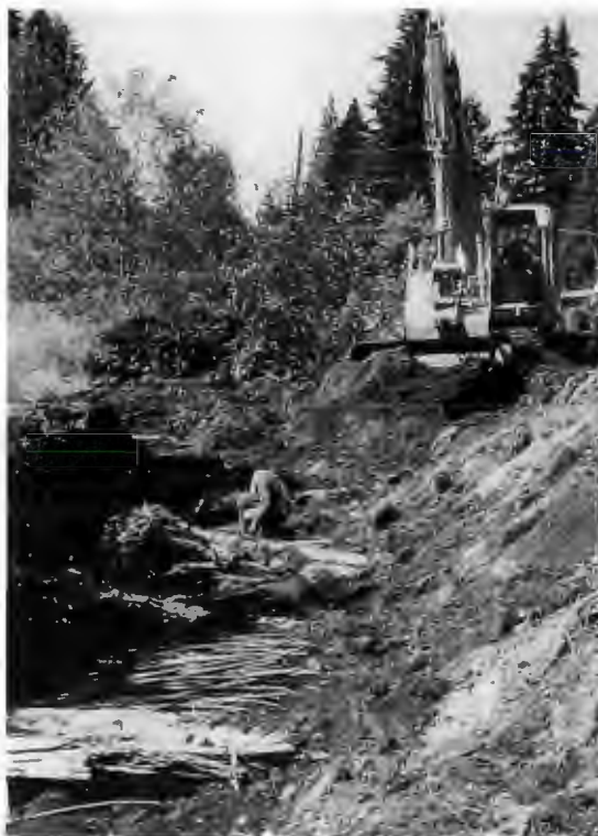
Figure 9.7: Backhoe in operation at a restoration site. Backhoes are mobile in rough terrain and can move rocks and logs with remarkable precision.
