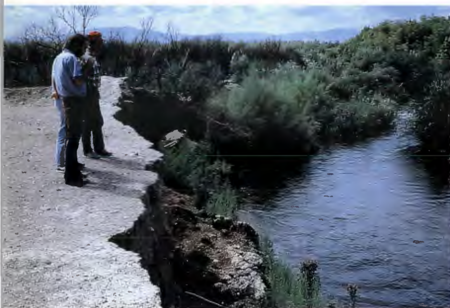
Figure 8.38: Eroded bank. Preliminary site investigation and analyses are critical to successful streambank stabilization design.
