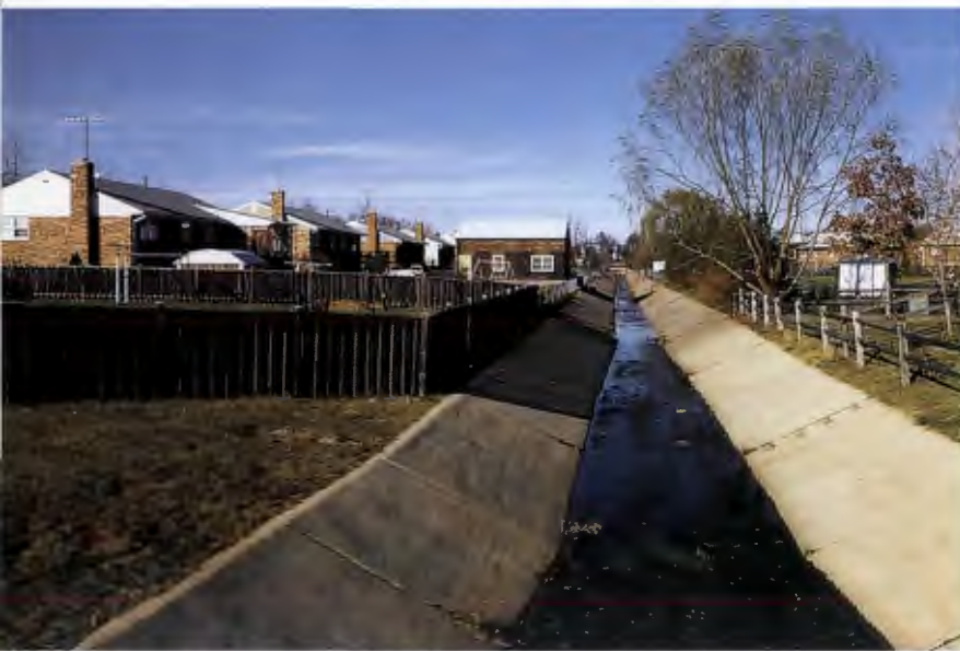
Figure 3.10: Stream channelization. Instream modifications, such as uniform cross section and armoring, result in ecological decline.
