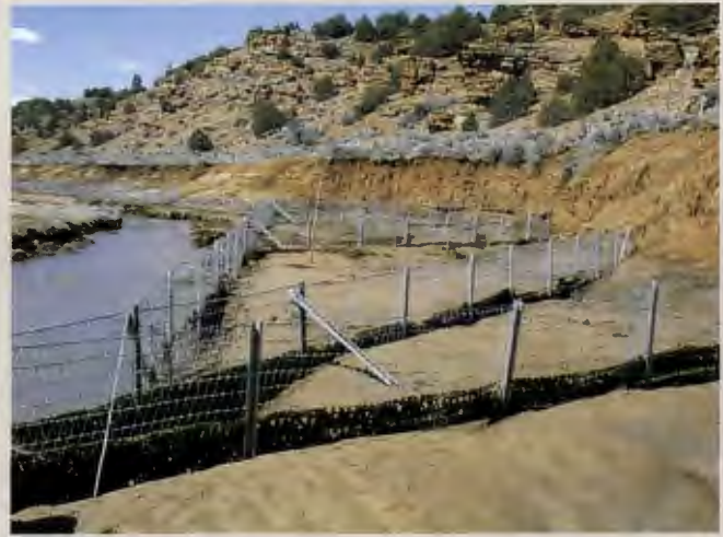
Figure 4.17: Recently installed treatment. (April 1987.) Porous fence revetment designed to reduce bank failure.
