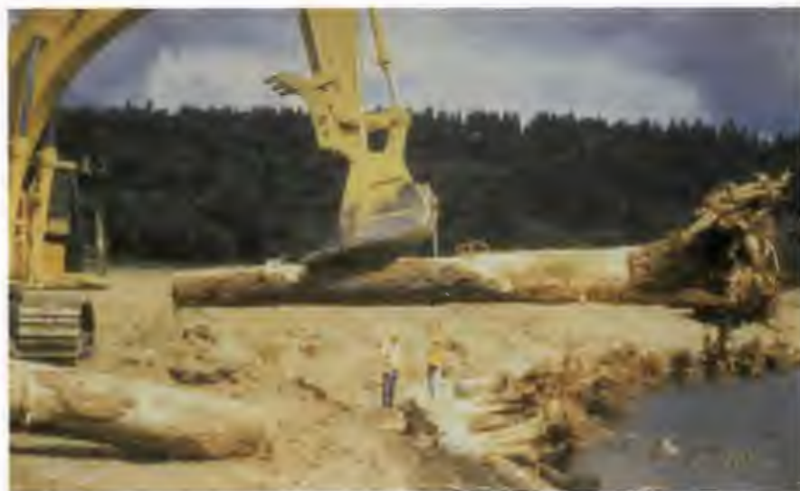
Figure 8.43: Installation of logs with intact root wads. An advantage to using tree revetments is the creation of habitat for invertebrates and fish along the streambank.
