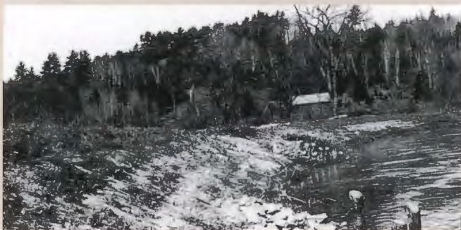
Figure 6.12: Brushmattress and plantings after spring runoff in March 1938. Note pole jetties. Brushmatting involves applying a layer of brush fastened down with live stakes and wire.
