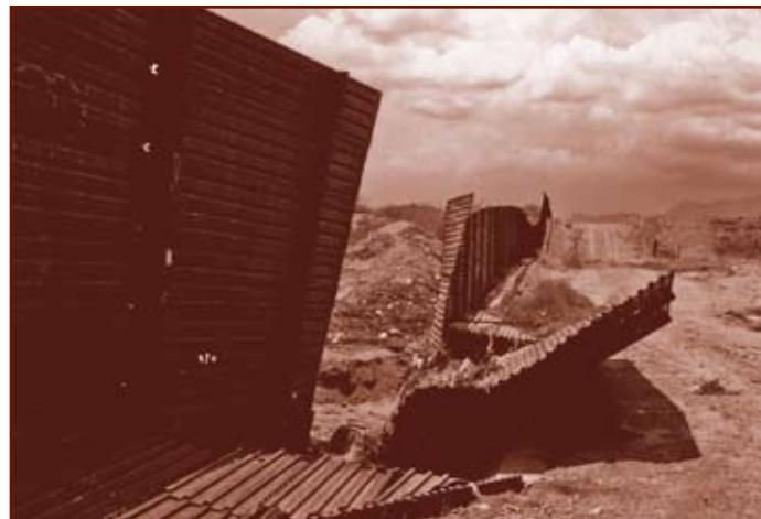
*Installation of security fencing without regard for environmental factors such as stormwater runoff may produce accelerated erosion and resulting instability. (Source: International Boundary and Water Commission)*
