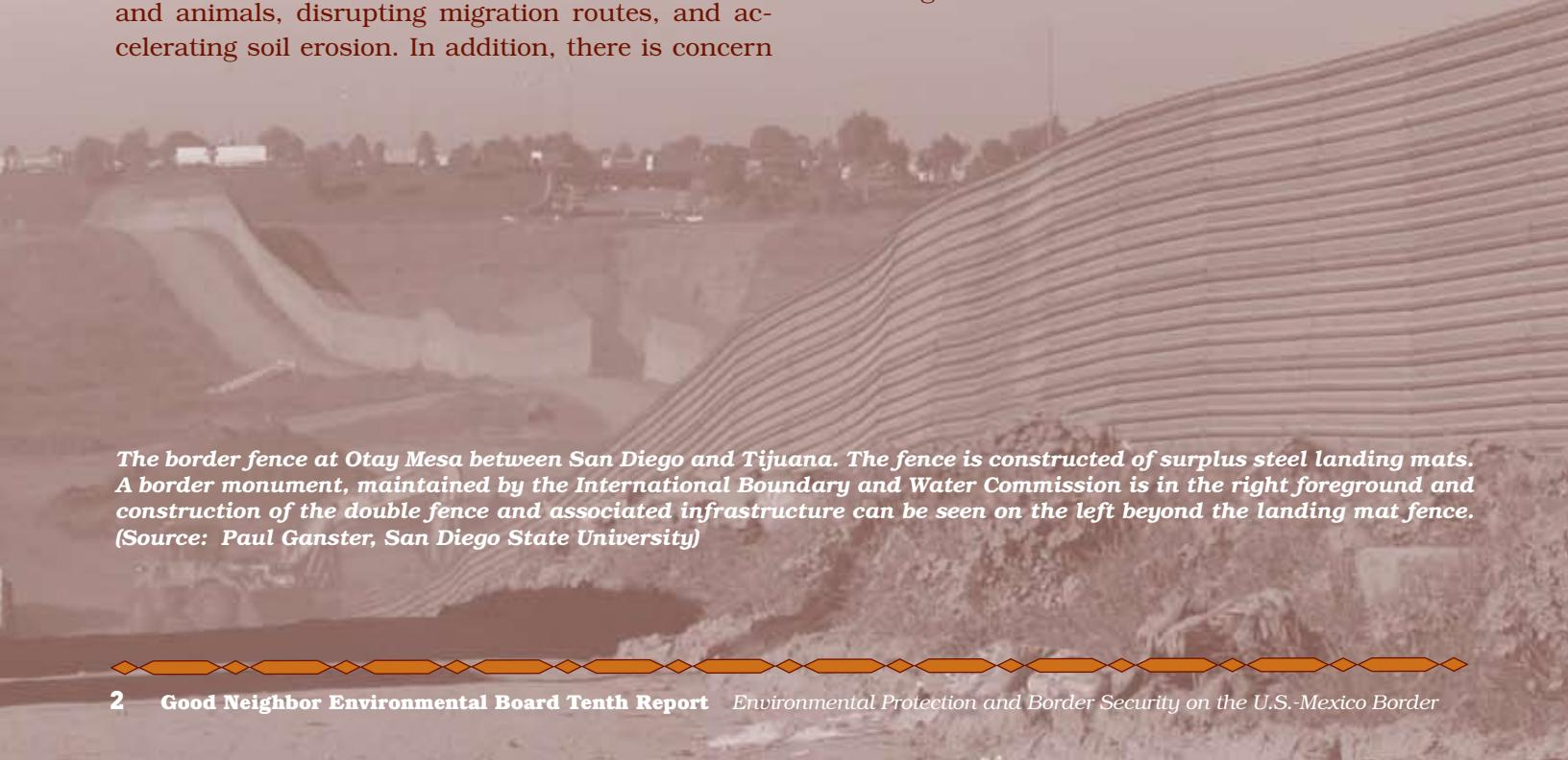
**The border fence at Otay Mesa between San Diego and Tijuana. The fence is constructed of surplus steel landing mats. A border monument, maintained by the International Boundary and Water Commission is in the right foreground and construction of the double fence and associated infrastructure can be seen on the left beyond the landing mat fence. (Source: Paul Ganster, San Diego State University)**
