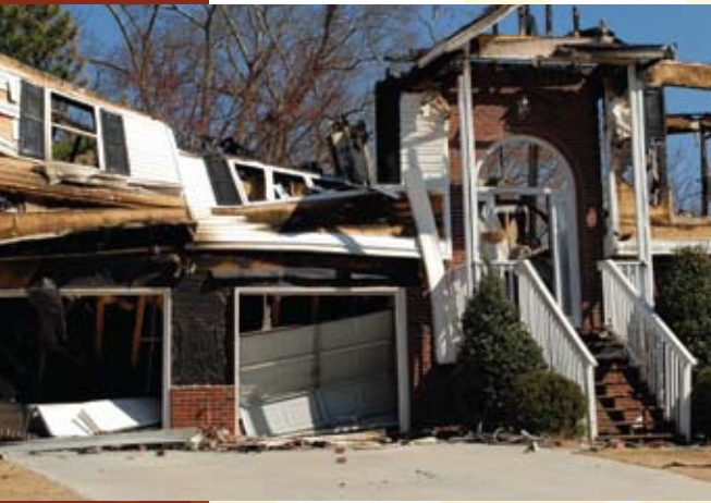
Explosion and fire damage caused by the volatile chemicals used in a meth lab.
