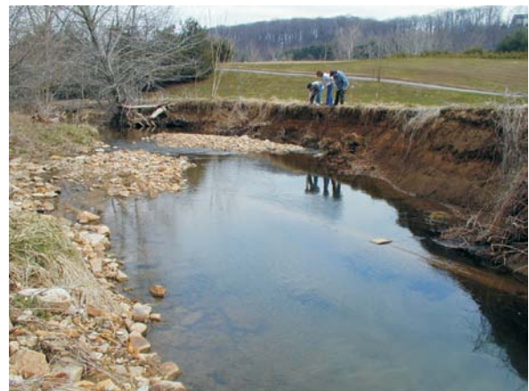
Figure 4. Incision and infrastructure exposure at Minebank Run before restoration.
