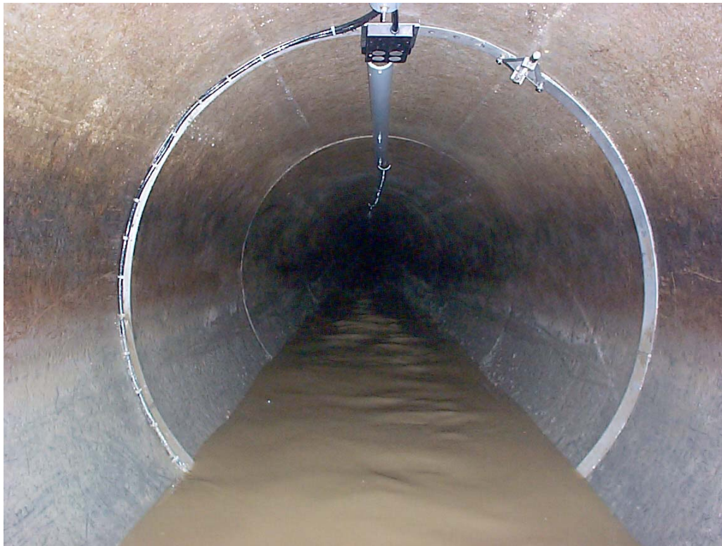
Figure 4-10. ADS 4000 flow meter components.
