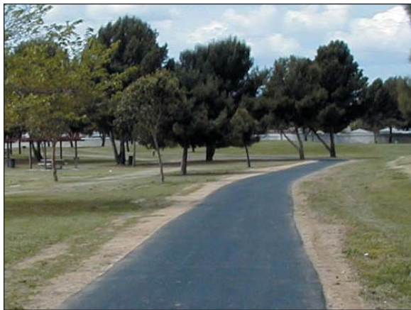
This walking path at the Earvin “Magic” Johnson Recreation Area in Los Angeles County is made from rubberized asphalt, which is more resilient than traditional asphalt.
