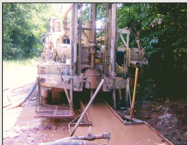
Figure 5. Drilling new, deeper residential well.
