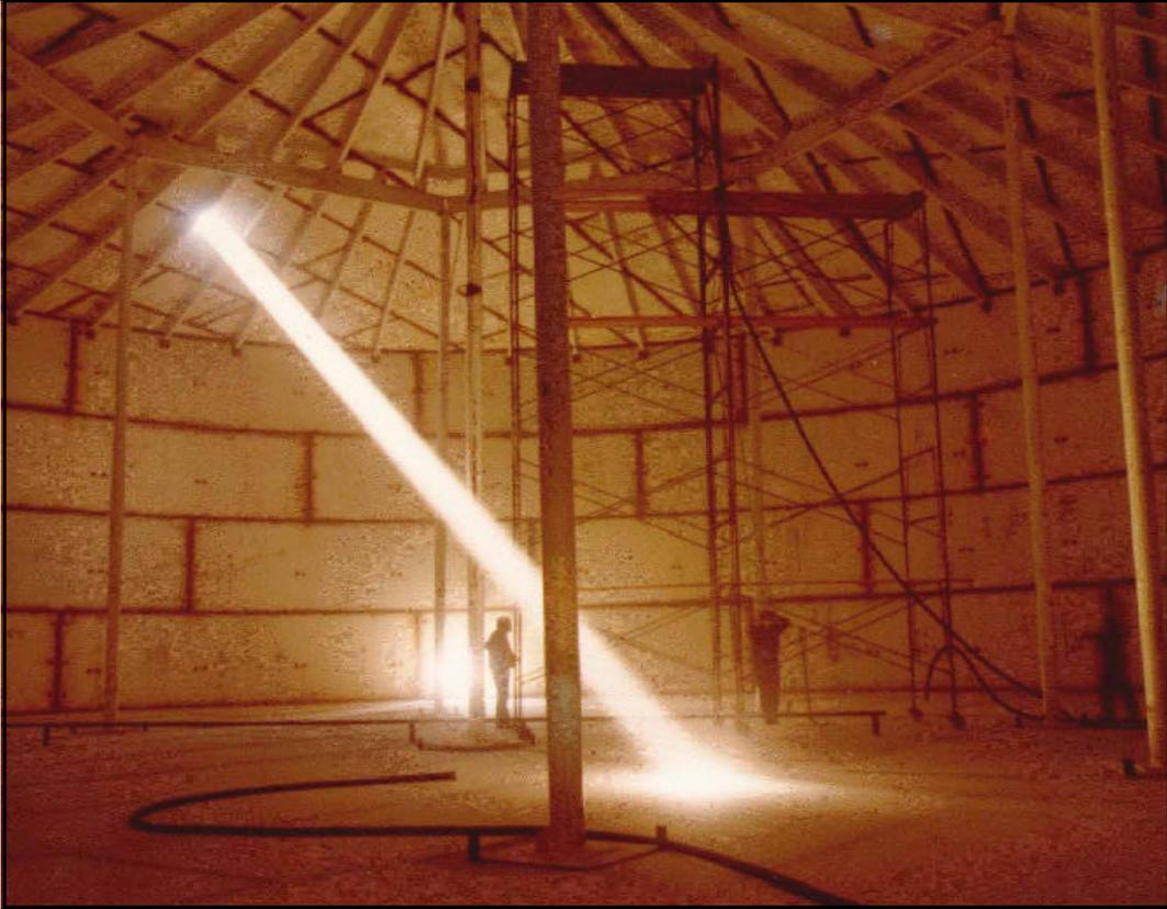
*The construction of a treated water storage tank nears completion in Nuiqsut, one of the most northerly communities in Alaska. In many Alaska Native communities, water tanks and treatment plants must be elevated on pilings to prevent the heated facilities from subsiding into the permafrost.*
