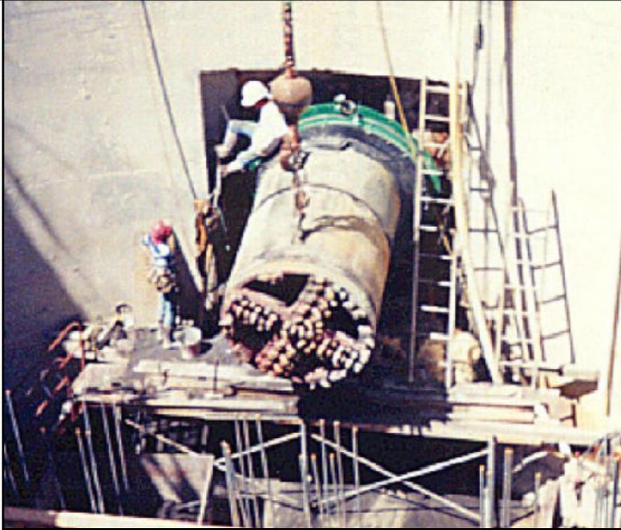
*Workers retrieve a tunnel boring machine (TBM) used to excavate an underground passage for a transmission line. TBMs allow water systems to bore through rock at rates faster than conventional drilling and blasting methods. By avoiding the need to tear up streets and set underground explosives, TBMs also minimize traffic disruption and noise for the surrounding areas.*
