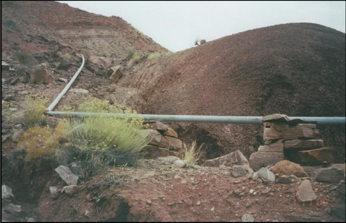
*The expense of burying pipe leads some systems to develop expedient but precarious solutions such as the one pictured here. Water service will be disrupted if pipes are not buried or otherwise adequately protected.*
