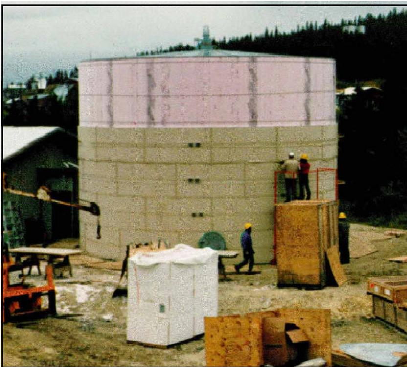
*A storage tank under construction in White Mountain, Alaska, is encased in insulation to prevent water in the system from freezing. Constructing water systems to withstand extreme weather conditions is one reason Alaska Native Village systems have high per-household needs.*
