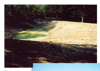
Sediment basins prevent excess sediment from reaching the lake by collecting runoff water and allowing sediment to settle out of the water and be deposited in the sediment basin.
