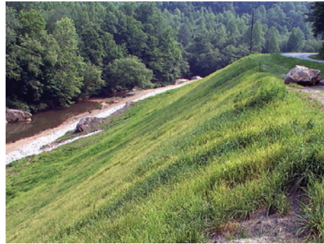
Rock Creek bank after restoration.
