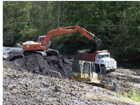
Bank restoration along Rock Creek has reduced sediment loading by 500 tons per year.
