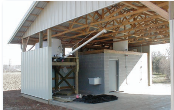
This chemical-handling facility replaced one that was directly adjacent to Mills River.
