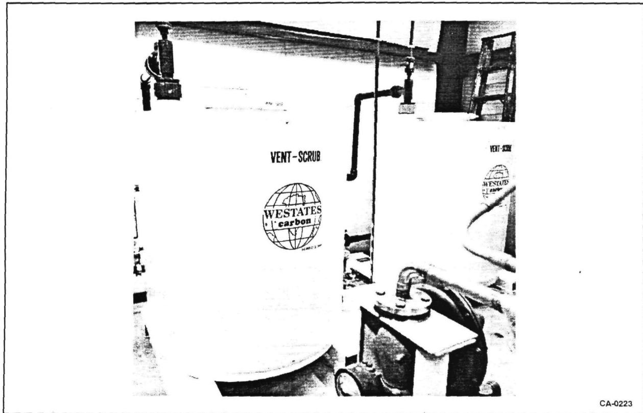
*Figure 3.1.4-3. High Capacity Hydrogen Sulfide Removal Tank Installation at Groton Landfill*
