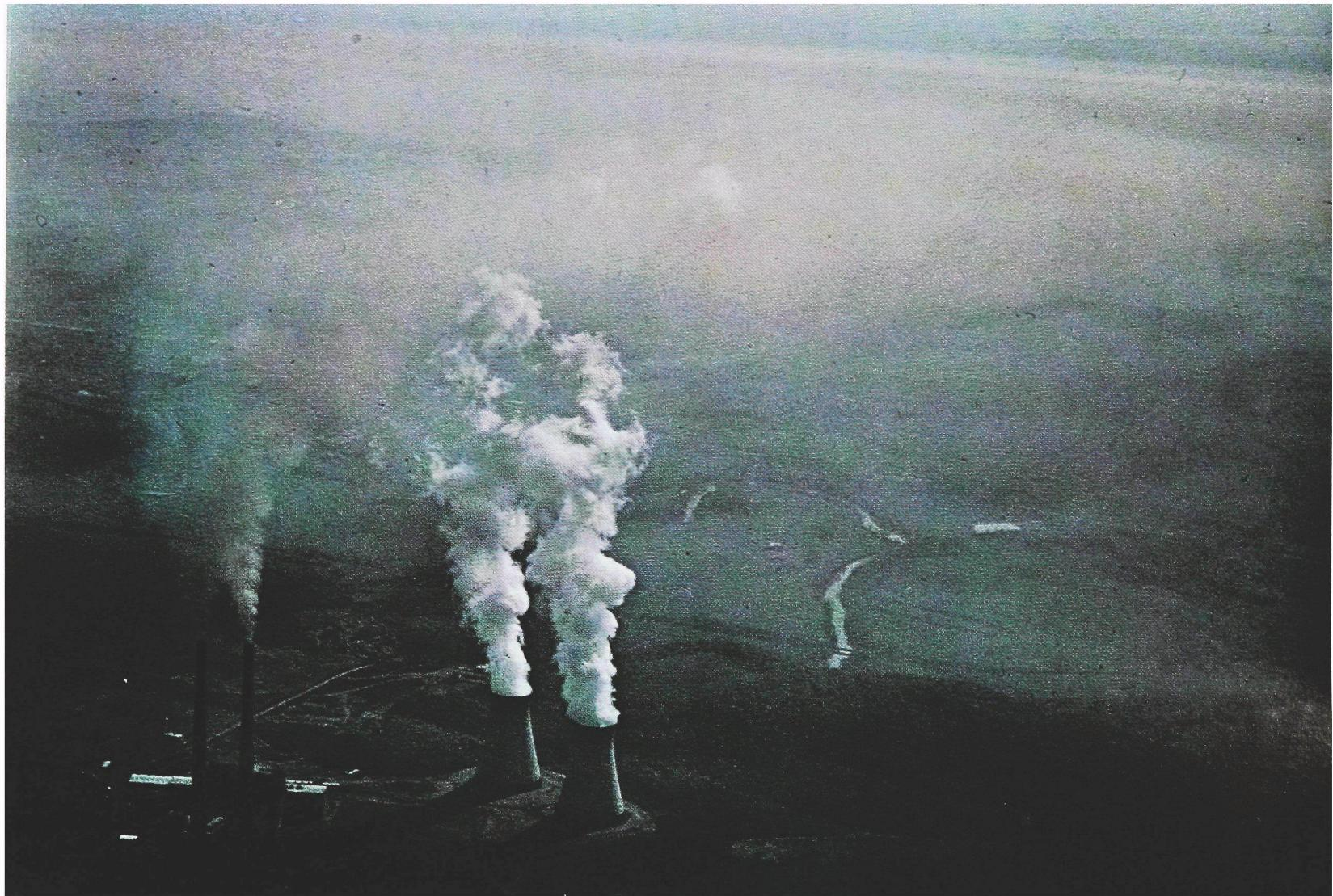
Plate 2. Homer City plume, May 4, 1970, 0838 EST. Visible plume accomplished by means of intentional, limited fly ash release.
