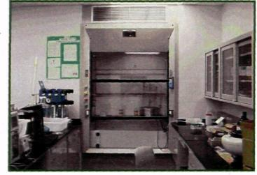
the laboratory by approximately 800 CFM. The estimated energy savings based on the use of these hoods, mostly from the energy needed to condition the replacement air, is approximately 920 MBTU per year and \$19,200 per year in energy costs. An additional five fume hoods will be replaced under this program over the next two years, with an additional projected savings of 800 MBTU per year and \$17,300 per year in energy costs.
