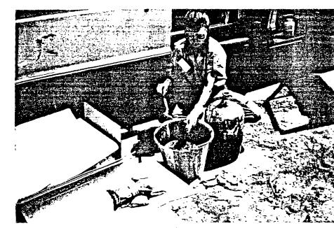
Photo 7. filling sludge sample jar from sludge composite
