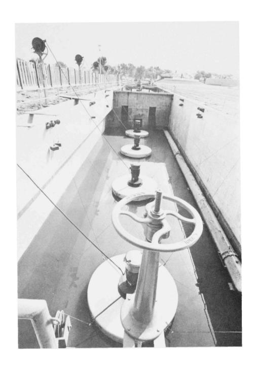
Figure 10. View of one stabilization tank compartment while empty. Floating surface aerators are shown at bottom of tank.
