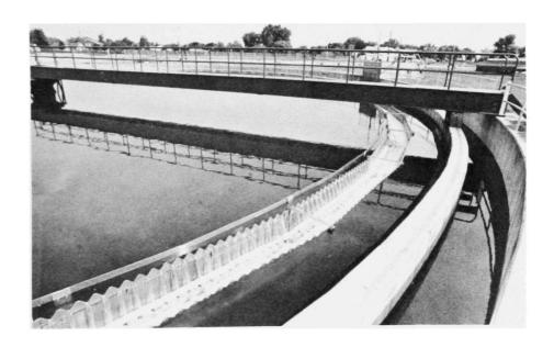
Figure 15. Detailed view of clarifier showing scum baffle, effluent trough, deflector skirt, and feed trough
