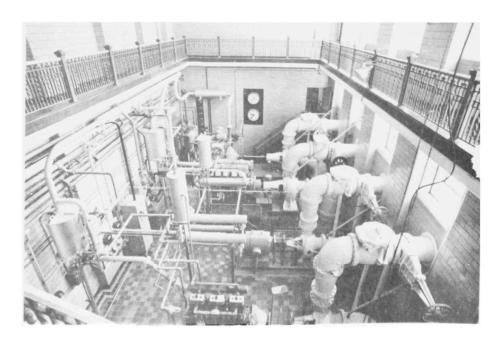
Figure 6. New gas driven engine and pump shown in relation to existing pumping facilities (new pump is at the top of photo)
