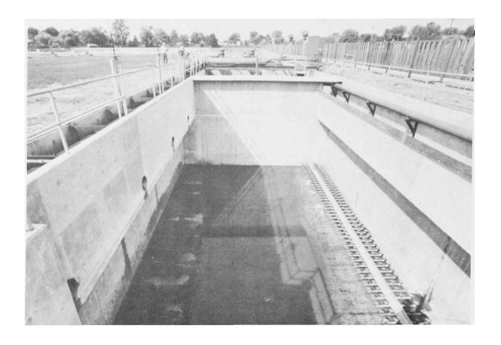
Figure 8. View of larger compartment of contact tank. Disperser system is shown at lower right and overflow weir at top right
