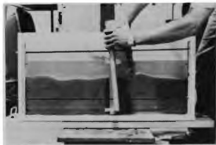
Figure 2 CGA Injection: Pilot Trough Test (Midway)
