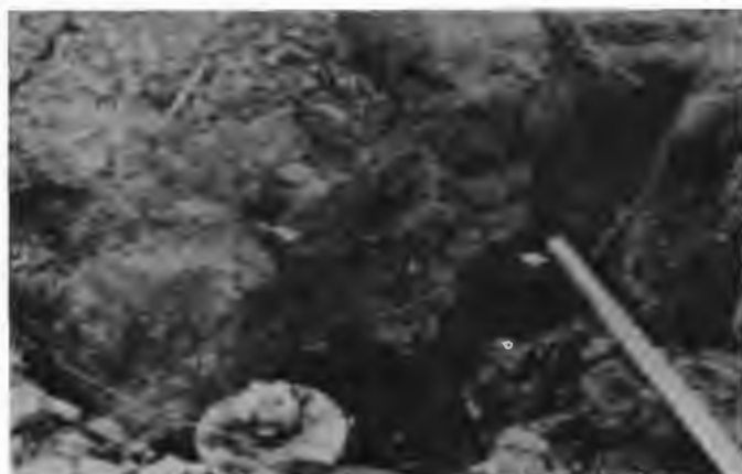
Figure 4 Concentrated Pesticide Runoff Collected in Interceptor Pits at Burn Site. Residues from pit 1 transferred to pit 2. Floating pump used to transfer runoff into 17H drums by personnel wearing full protective clothing.
