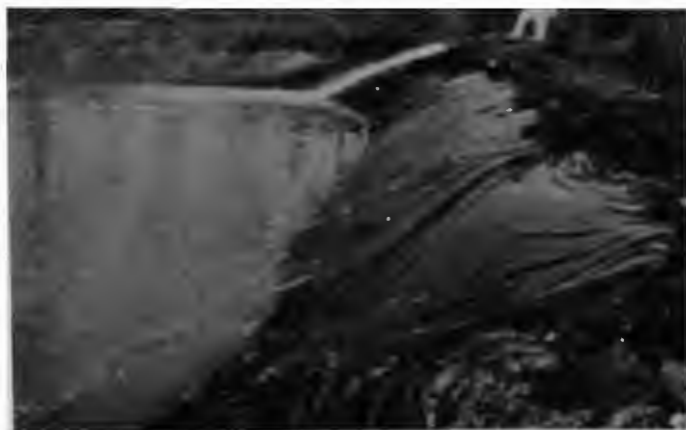
Figure 3 300,000 Gallon Treatment Lagoon Containing Contaminated Runoff from the Creek. The lagoon was lined with 24 mil Visqueen with side slopes of 1.5 to 1. Pumping station transferring creek to treatment lagoon, final grade lagoon apron.
