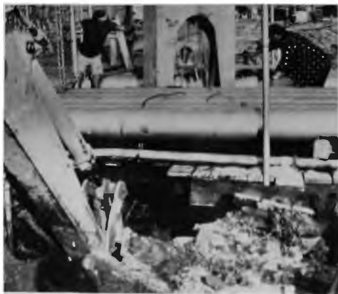
Figure 4 Working in Confined Area with Backhoe and 9-Ton Clamshell
