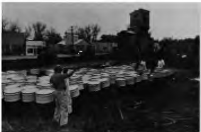
Figure 7 Contaminated Residues Packaged in 17H Drums. 485 Drums Were Loaded Using Front-end Loaders and Transported by Covered Trucks for Ultimate Disposition.
